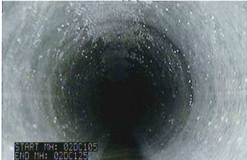
Same location after pipe lining
