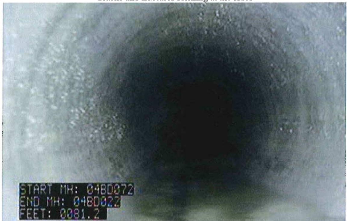
Same location after pipe lining
