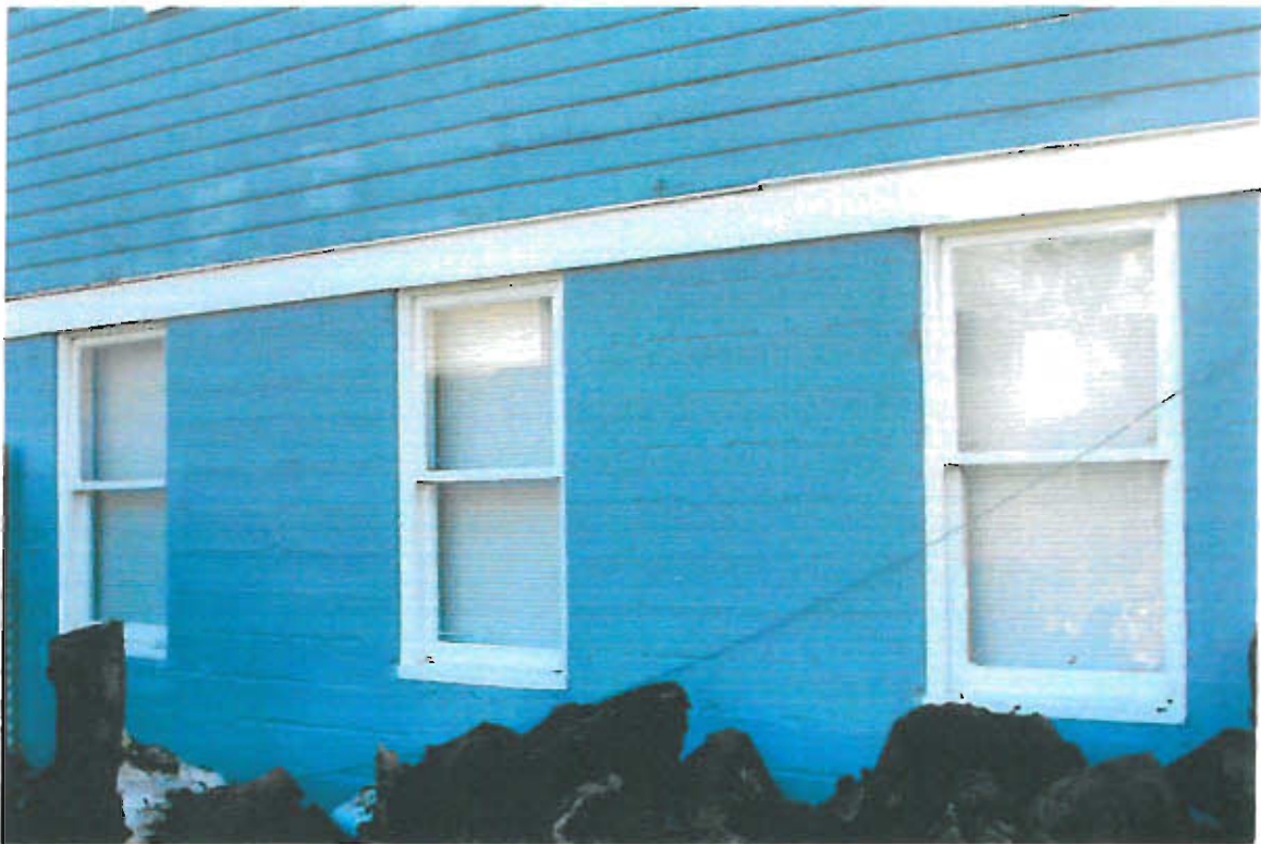
3 basement windows replace
