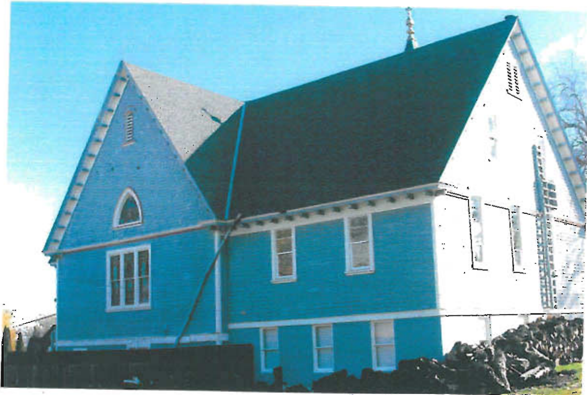
3 windows - basement replace Rear
