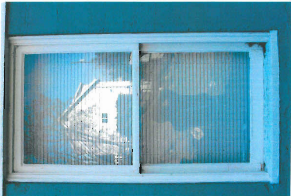
Rear-basement replace 3 windows
