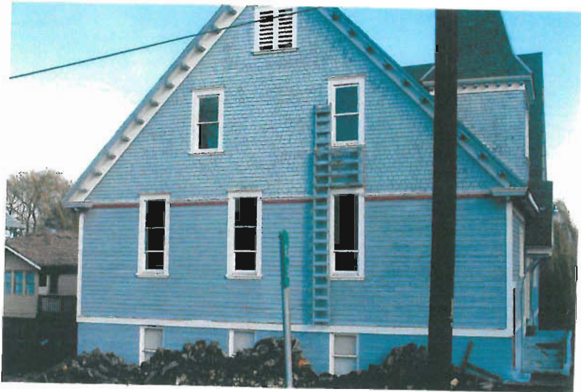
3 basement windows side
