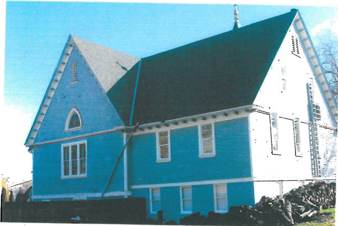
3 windows - basement replace Rear
