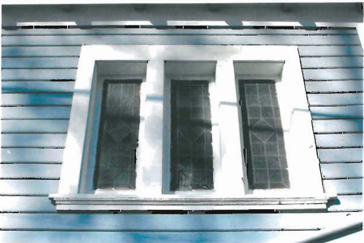
repair stained glass
