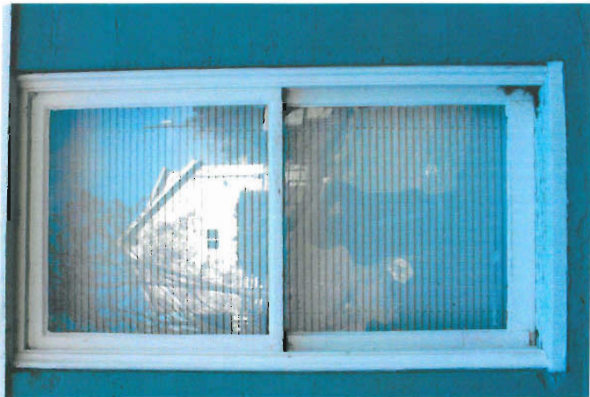
Rear-basement replace 3 windows
