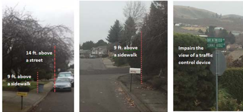
City of The Dalles Municipal Code 11.20.020 regulating street trees requires all trees growing near a sidewalk street or alley to be trimmed so that the limbs and branches are not less than nine feet above the sidewalk and 1) feet above the street. These trim requirements allow safe passage for pedestrians on sidewalks as well as garbage trucks and school buses traveling on streets and alleys.
